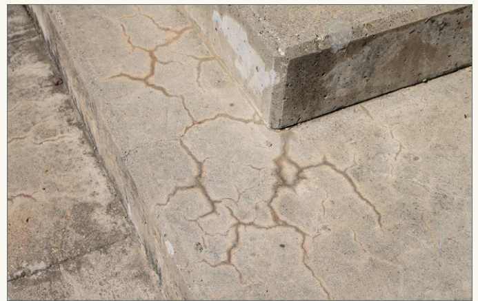
Figure 1: Effects of ASR on a Concrete Structure
