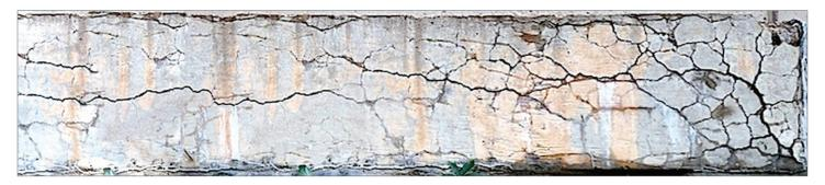
Chemical attacks on concrete refer to the deterioration and damage caused by various chemical substances that react with components of the concrete. These reactions can compromise the integrity, strength, and durability of concrete structures. One of the most common types of chemical attacks on concrete is sulfate attack.
