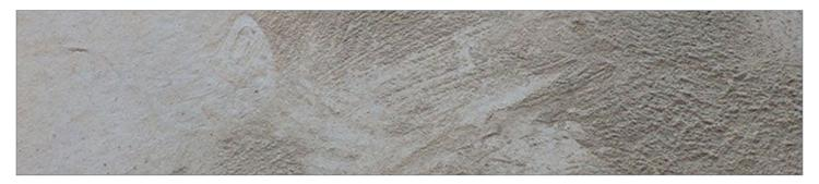
"Dusting" is when the surface of hardened concrete breaks down into a loose powder. This is also sometimes referred to as "chalking." These surfaces are easily turned into powder under any kind of traffic and can be scratched easily.
